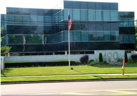
490 Wheeler Road - Hauppauge, NY
