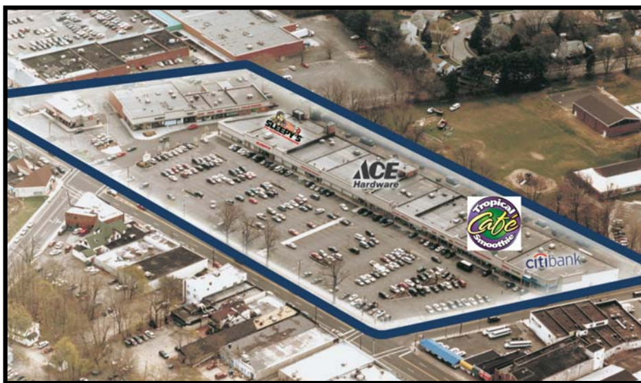
The Village Commons - 32 E Main St, Smithtown
